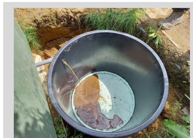
Dewatering box in operation
