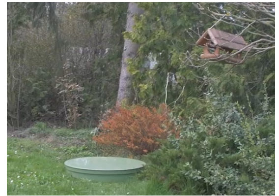
WWTP TOPAS S 5 after installation
