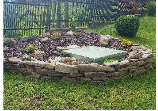
WWTP TOPAS S 8 after installation
